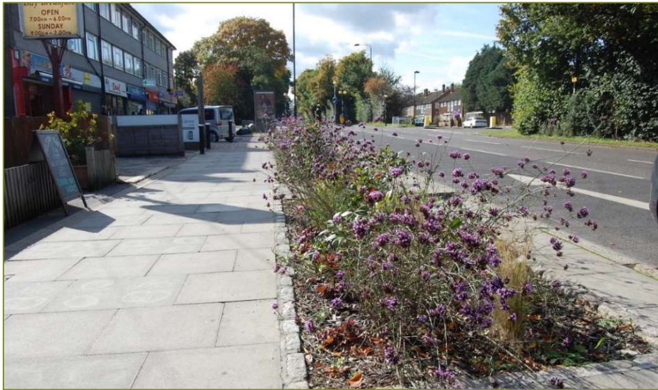
Figure 30: Rainwater gardens in Oakwood, Enfield, part of the SuDS network (source: Enfield Council)
