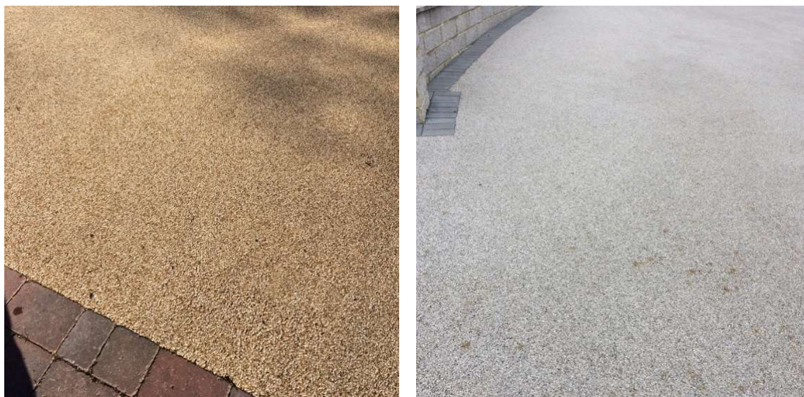
Figure 11: Examples of impermeable hardstanding (source: Google Images)
